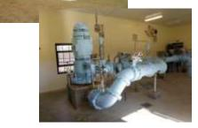
Two ASR wells in two different aquifers within a single wellhouse
